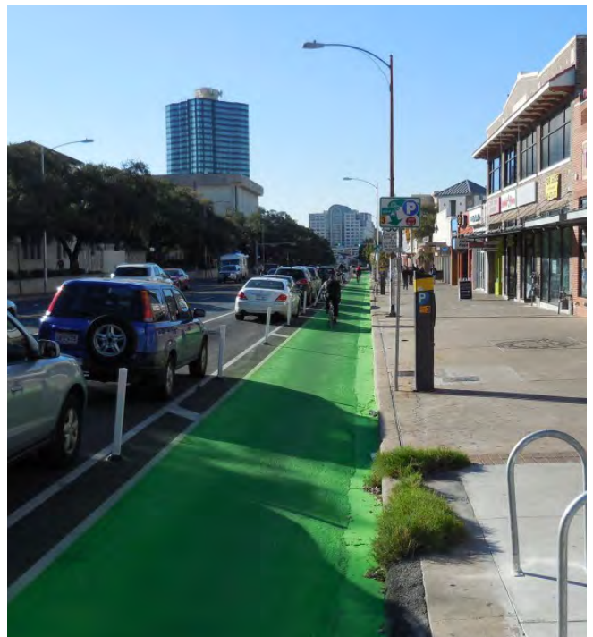
PROTECTED BIKE LANE IN AUSTIN, TX
