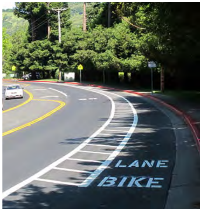
BUFFERED BIKE LANE IN FAIRFAX, CA (SOURCE: NACTO)
